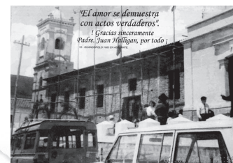
1968 - Finally! We've started the building
